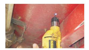
9. Drilling upward from underneath the header, use the 3/8" drill bit supplied to drill thru the metal trough and poly liner as illustrated. Drill at the lowest point in the trough. Install a 1/4-20 x 1 1/4" fanged elevator bolt in each hole before drilling the next hole.
