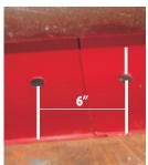
15. With the panels wedged and properly gapped at each joint, finish securing each panel as was described in Step 11. Use the Recommended Hole Location as illustrated on the following page. Install a 1/4-20 x 1 1/4 fanged bolt in each hole before drilling the next hole.
